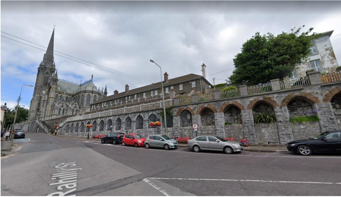
Figure 4. 7 Saint Colman's Cathedral Buttresses (19)
