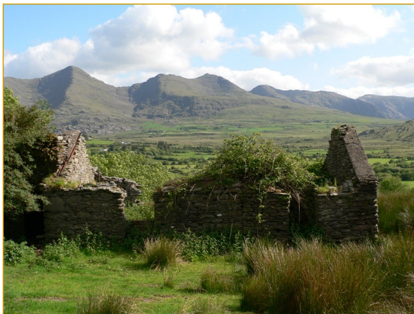
Abandoned farm building in Keas, Glencar
