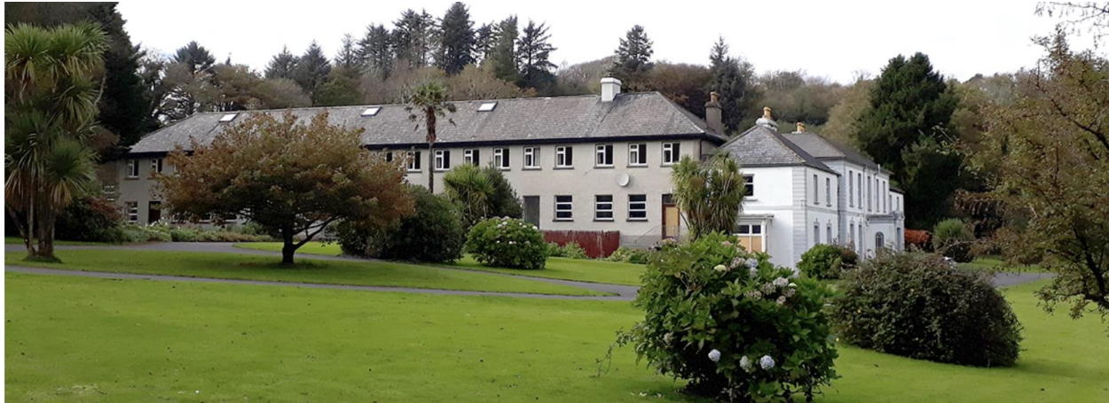
Figure1: View from East of Myross Wood House in County Cork, a demonstrator in the Energy Pathfinder: Towards Zero Energy for Historic Buildings research programme. To the right, is the original entrance wing facing North-East, to the left is the 1950's reconstructed wing facing South East.
