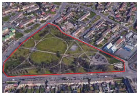
Figure 2.5: Ariel photograph of Gerry O'Sullivan park
