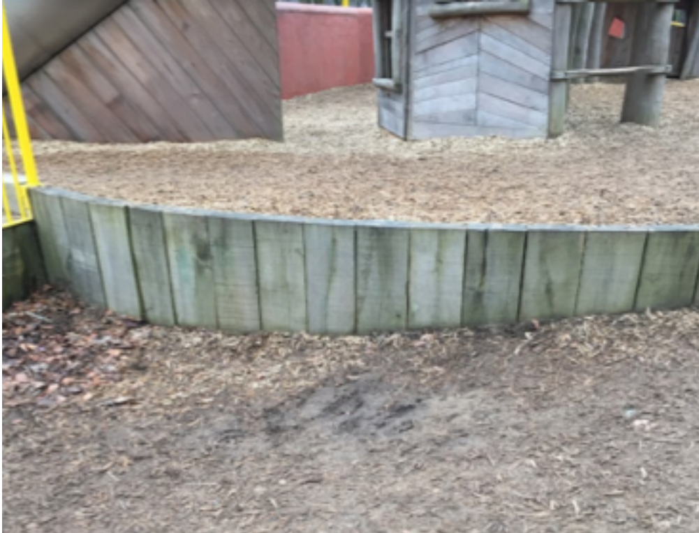
Figure 6.6: An example of poor visual contrast between paths and changes in height in Fitzgerald's park
