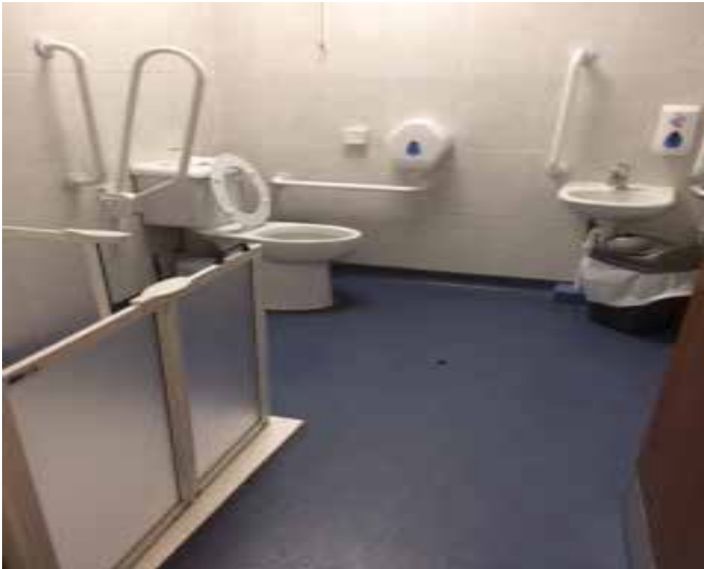
Figure 6.10: An example of toilet facilities located in community centre in Tory Top park
