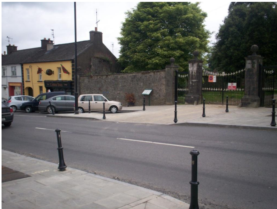
Fig. 16: Gate opening onto the main street of Doneraile for Doneraile Court. Gate known locally as 'The Lord's Gate.' Source: http://homepage.eircom.net/~neillod/tomos.html accessed on 14 September 2013
