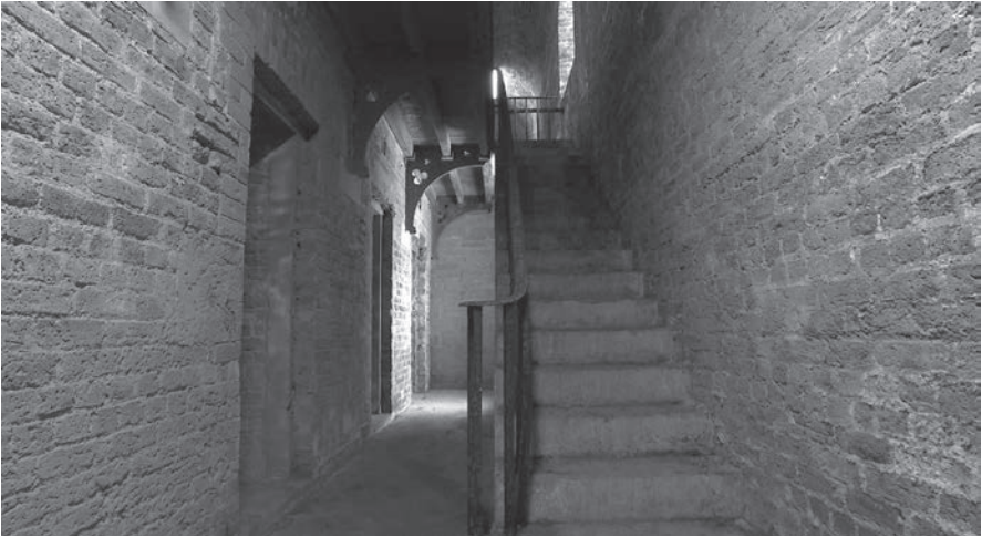
Figure 15.1 Interior of the Punishment Block with the stairs to a mezzanine landing. There were 18 cells on the two storeys of this main wing and six more in a single-storey corridor at a right-angle to that pictured. The walls would have been whitewashed in the 19th century, but this was removed in the 1980s. (Image © authors)
