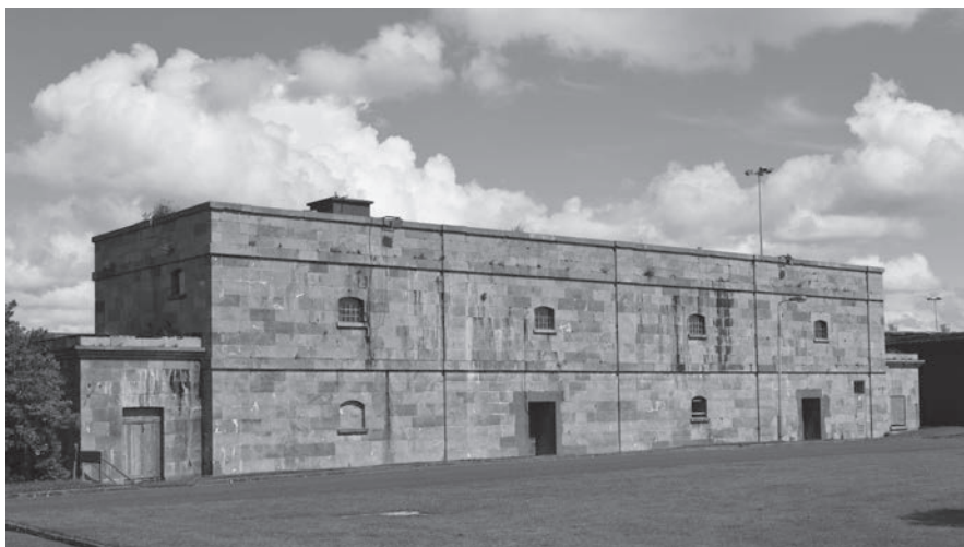
Figure 11.1 The façade of the Punishment Block, completed in 1860, before its recent restoration. (Image © authors)
