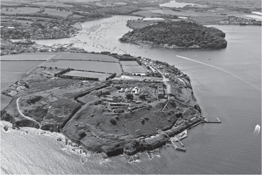
Figure 6.4 Fort Camden from the east. (Image © Cork County Council)
