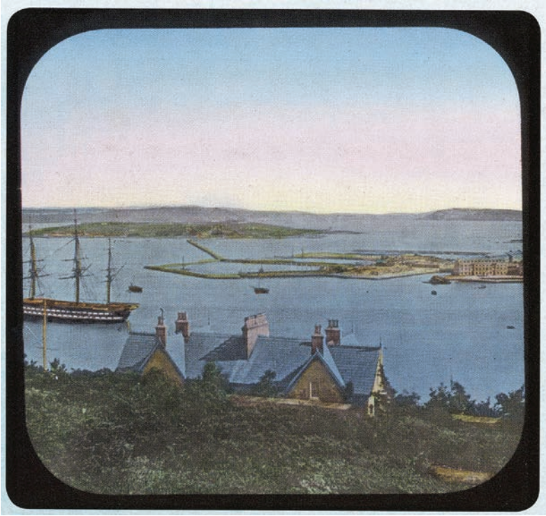
Figure 14.2 Hand-tinted, late 19th-century lantern slide of Spike and Haulbowline islands and the connecting causeway, completed in 1867. Construction was underway on the coffer dam and landfill on the extension to Haulbowline. (Image © courtesy of Collection of Michael Lenihan)
