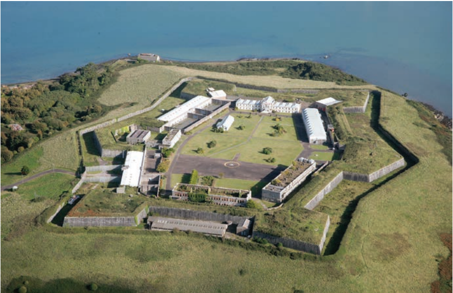
Figure 18.1 Aerial view of Fort Mitchel, Spike Island, taken before the renovations carried out in 2016. (Image © courtesy of National Monuments Service)
