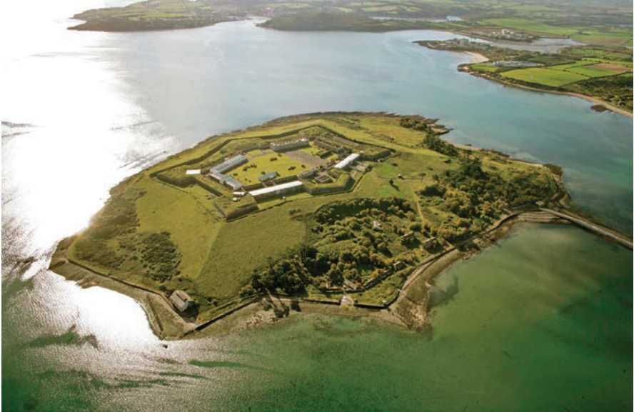
Figure 10.1 Spike Island from the north, note the artificial slope of the glacis. (Image © courtesy of National Monuments Service)
