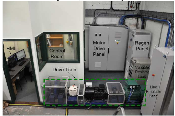
Figure 2 Test Rig and Control Room
