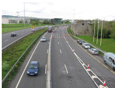
Figure 8 – Traffic Management Provided during Rehabilitation
