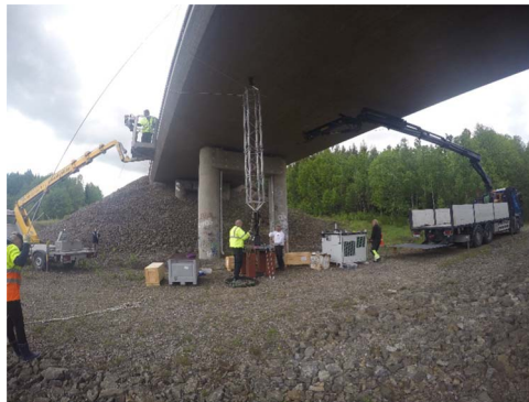
Fig. 3. Photograph of shaker for providing excitation to Pershagen Bridge.
