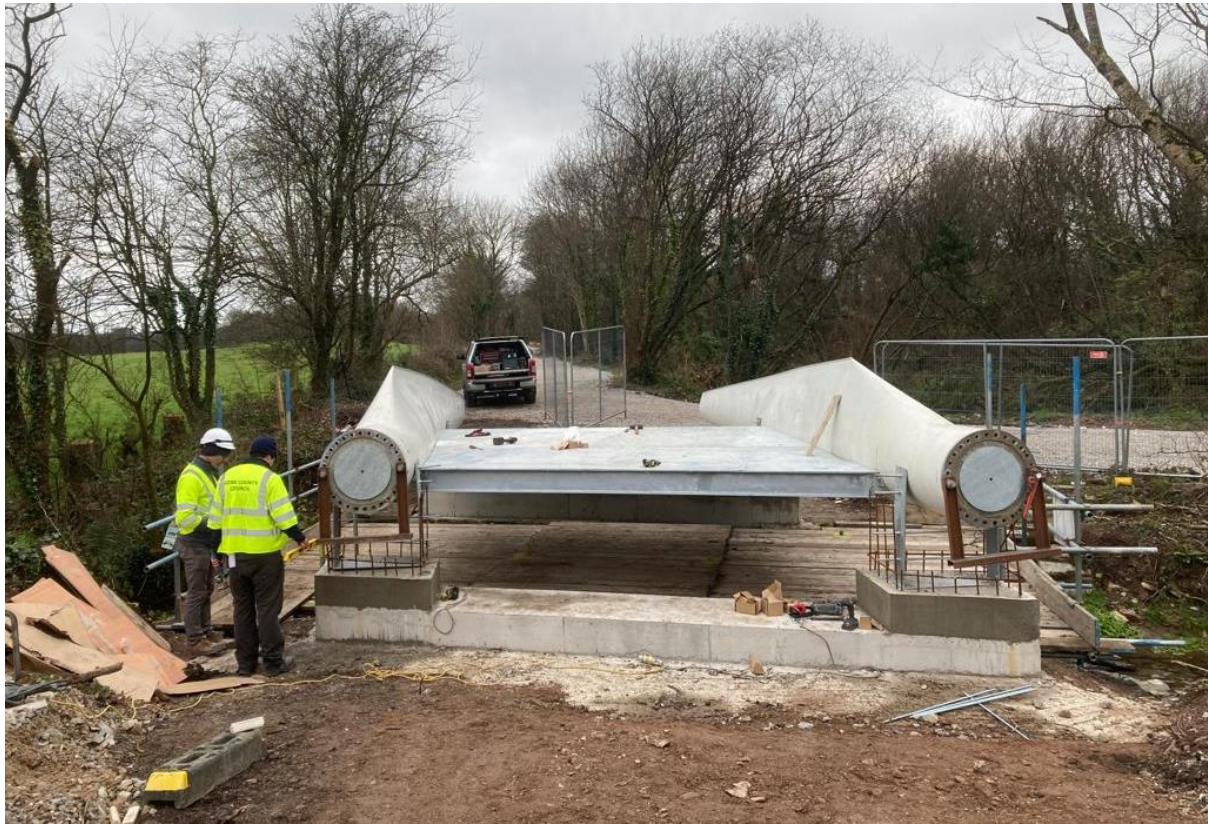
Figure 6.2 The BladeBridge installation near the Midleton train station in Cork, Ireland, under construction late January, 2022 (source Author)
