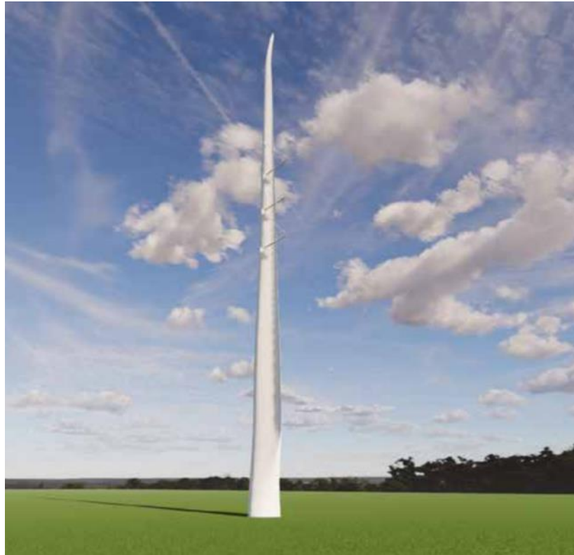
Figure 2.12 Re-Wind ‘BladePole’ transmission line design concept (McDonald et al., 2021)
