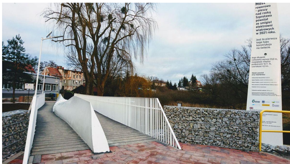
Figure 2.5 Anmet pedestrian bridge in the town of Szprotawa (Stone, 2022)
