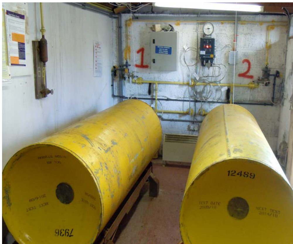
Figure 8.1: Part of the chlorination system of water treatment works.
