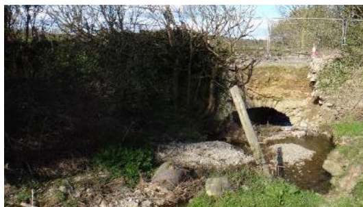
a) Upstream elevation of the bridge
