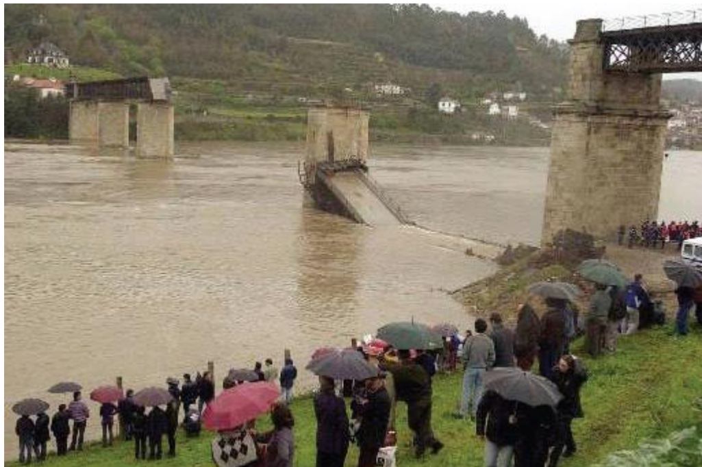
Figure 11.8 Collapse of Hintze Ribeiro Bridge in Portugal [98].
