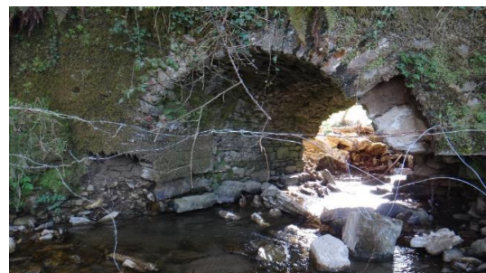
b) downstream elevation of the bridge
