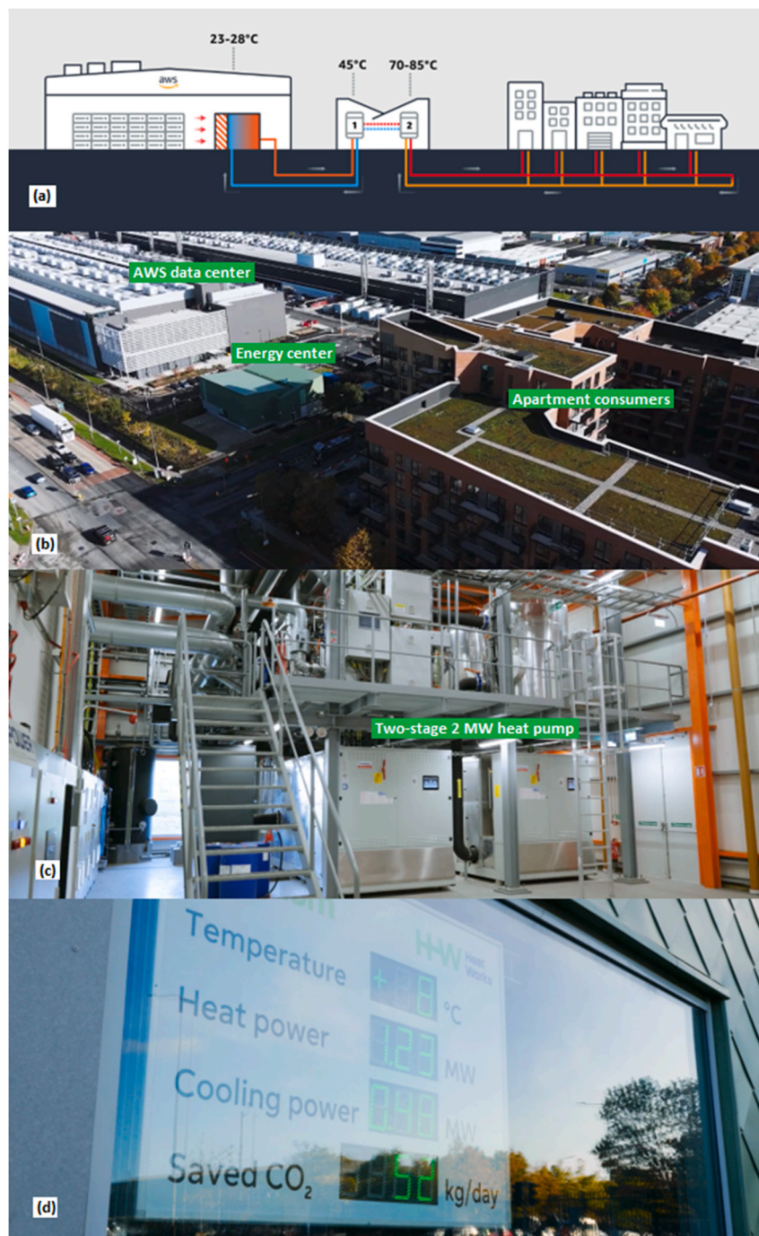
Fig. 25. Tallaght District Heating: (a) schematics of data center, heat pump, and consumer integration, (b) outside photograph, (c) one of the heat pump units in the energy center, (d) real-time monitoring and measurement for one of the units in a summer day.
