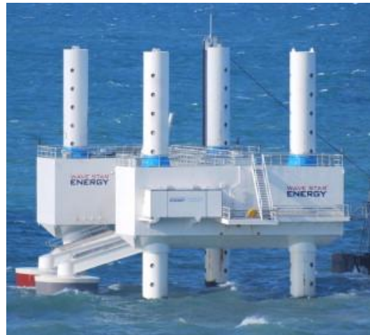
Fig. 1.2: Prototype of the Wavestar multi-body heaving WEC [21].
