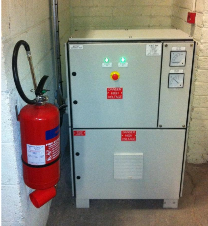
Figure 5.9: Front view of the high voltage battery enclosure including panel with associated control electronics
