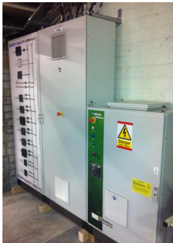
Figure 5.12: Microgrid panel and Triphase panel installations
