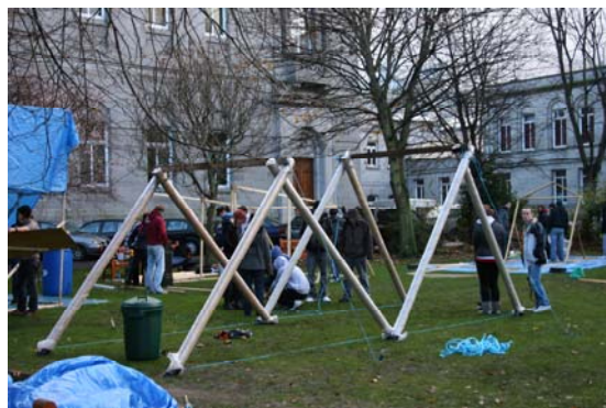
Figure 2 - Construction of ‘The Cardboard Cradle’, a design which incorporated recycled cardboard tubes from cardboard manufacturers
