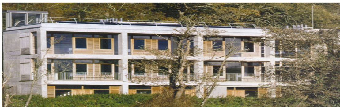
Figure 9.1: South Faade of the ERI Building at University College Cork, Ireland
