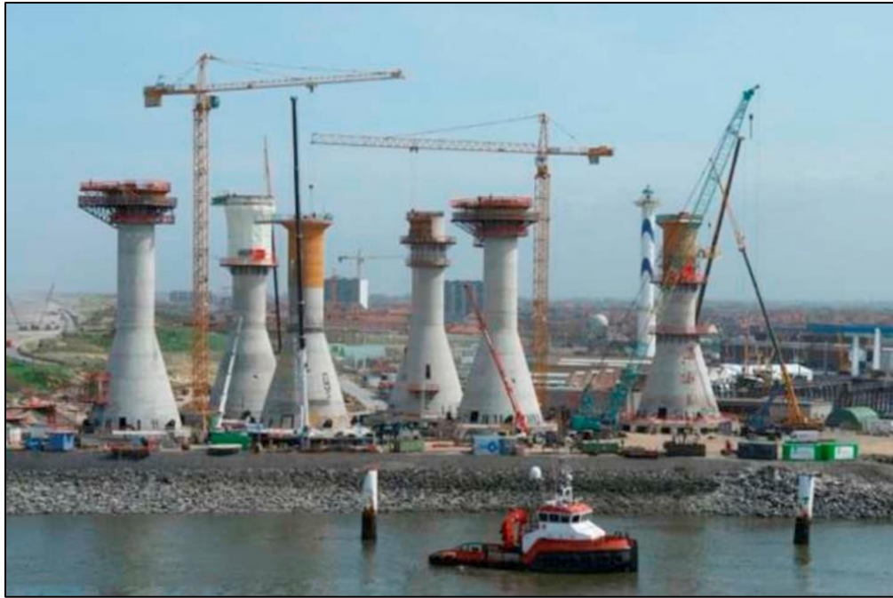
Figure 2-6: BAMs concrete GBFs prior to installation on Blyth wind farm. Source: (Esteban et al., 2015)
