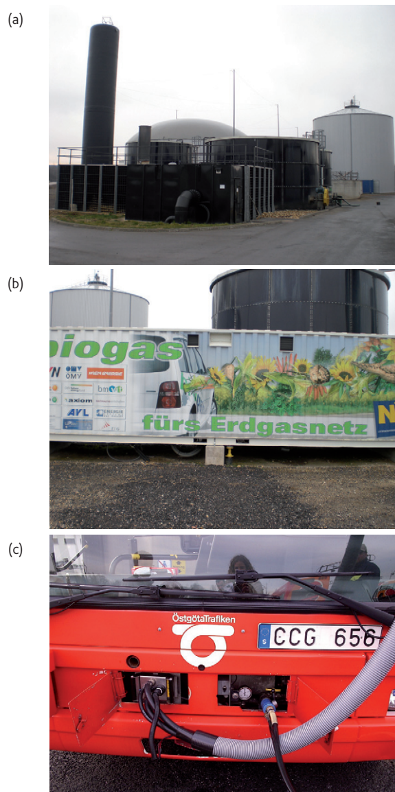
Fig. 3 (a) Facility producing biomethane from waste food in Austria. (b) Upgrading of biogas and injection of biomethane into the natural gas grid (yellow valve centre of picture) in Austria. (c) Injecting biomethane into a bus in Linköping, Sweden.
