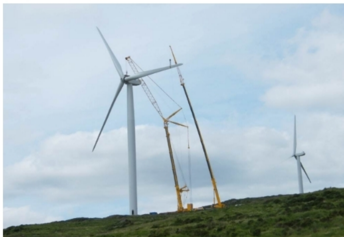
© Tony McGinley. SWS wind turbine being constructed, Kilgarvan, Co. Kerry, 2009.
