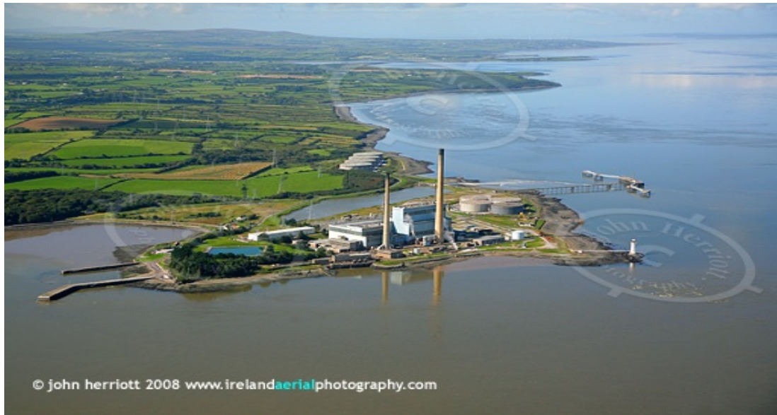
Figure 6.1 Aerial photograph of Tarbert Island, Co. Kerry. Note the ferry port to the left of the electricity power station in the centre foreground. This image highlights the disparate nature of development along the Shannon Estuary, with areas of intense industrial activity, the power station and ferry terminal in the foreground, interspersed into a largely rural mixed-use landscape (Source: © John Herriott).
