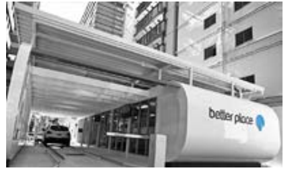
Figure 2. Battery Swop Drive-in Station
