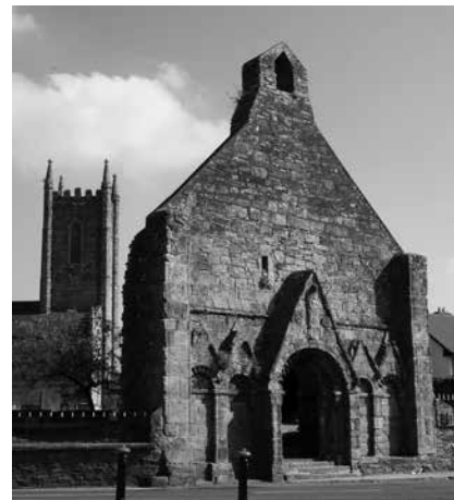
17. The west façade is all that survives of Roscrea Cathedral (c. 1130s).
