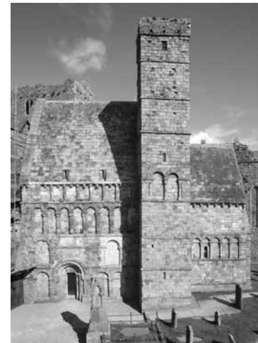
3. Cormac's Chapel, Cashel (c. 1134) from the south.
