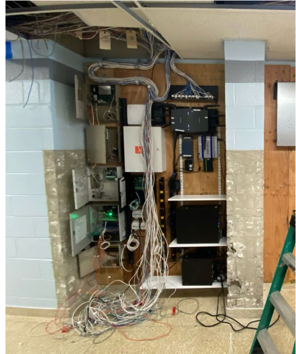
Figure 22 — (a) Employee Opens Office Door with Badge [6] ; (b) Access Control Installation in a Public Building in NYC [7] showing cables required
