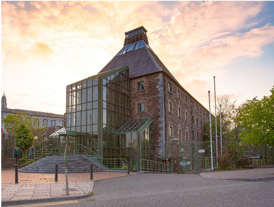
Picture 1: HEINEKEN Ireland, Leirim Street, Cork
