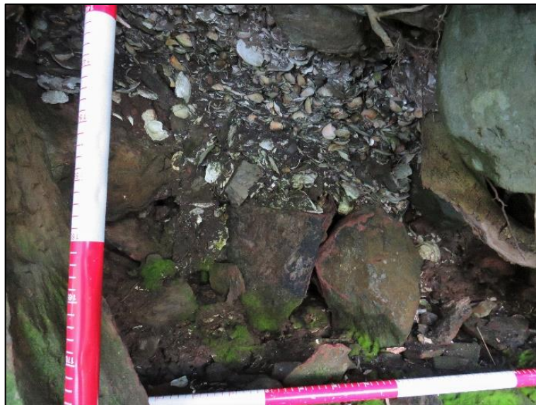
Figure CO.18: Shell deposit in section face in 2019.
