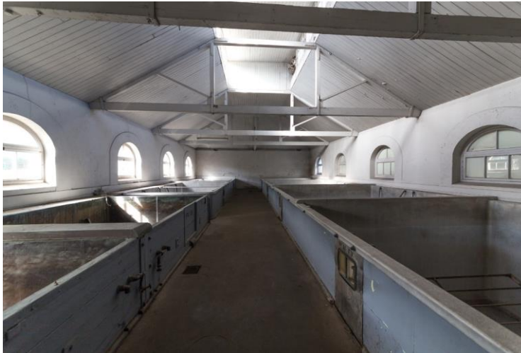
Plate 6.9. Upper floor of the fermenting block, the St. Mary's Brewery, Waterford. The two fermenting squares in the left foreground are original, dating to the brewery's renewal in 1899-1901. The remainder are mid-to-late-20th century replacements.
