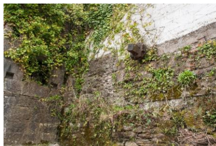
Plate 7.6 Partially surviving water-wheel pit and axle, Walker's Brewery, Fermoy, county Cork.
