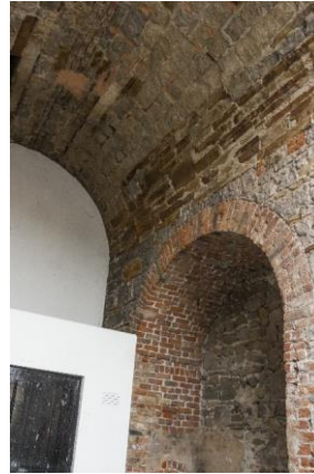
Plate 4.11. Vaulted ground floor of maltings with furnace arch at the St. Mary's Well Brewery, Carlow town.
