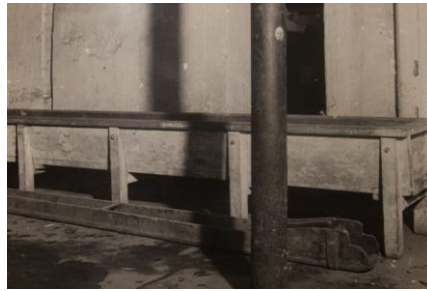
Plate 6.5. Cleansing stillion at the Millpark Brewery, Enniscorthy in 1957 (courtesy D. Lett).
