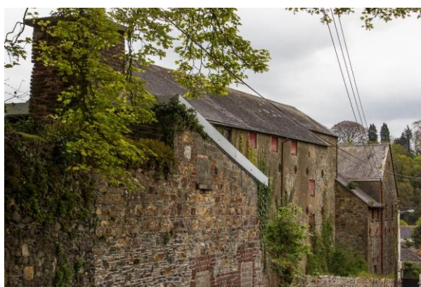
Plate 7.16 Engine house and chimney, dating to the mid-1860s reconstruction, on left. The chimney has been truncated and the engine house directly adjoins the truncated former brewhouse, in centre. The Millpark Brewery, Enniscorthy, county Wexford.
