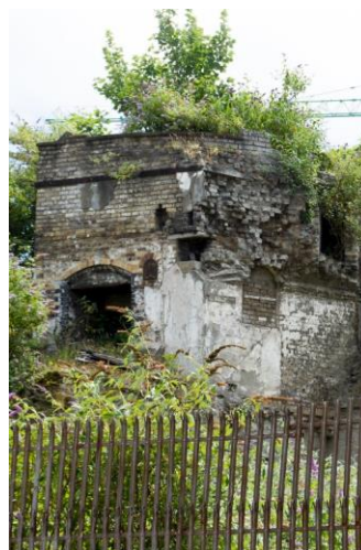
Plate 5.18. Brick setting for brewing copper, Watkins' Brewery, Dublin.
