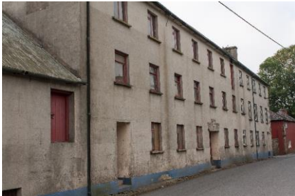
Plate 4.17. Barley stores, dating to the late-18th or early 19th century, at the Watergate Brewery in Bandon, county Cork.
