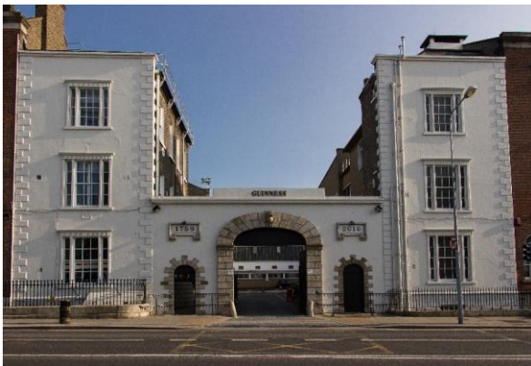
Plate 8.32. Decorative gateway and gate lodges, providing access to the 'north deck' of Guinness's Brewery, Dublin city. The buildings appear to date to the early 19 th century, having been depicted on the 1820 plans of the brewery.
