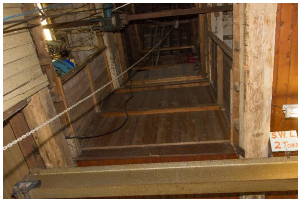
Plate 4.19. Full-height internal void, viewed from the ground floor, at the eastern maltings, Rutland Street, Cork city. The chain visible in the left foreground hangs from a hand-dressed timber sack hoist, reinforced by a steel H beam.
