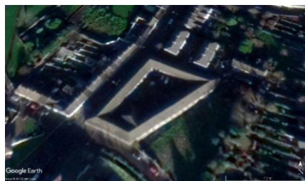
Plate 4.26. Aerial view of a courtyard maltings on King Street Upper, Wexford town. Source: Google Earth.
