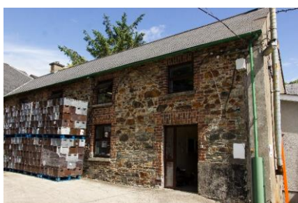
Plate 8.22. Simple office building at the Mill Park Brewery, Enniscorthy, county Wexford. Constructed in the mid-1860s redevelopment of the brewery.
