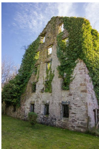
Plate 7.2 Multi-storey flour mill, Grubb's Brewery, Clogheen.
