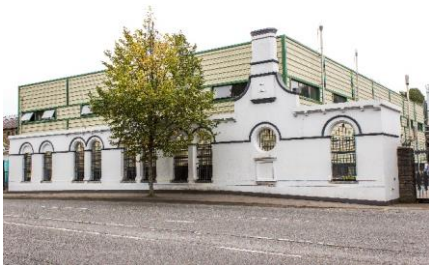
Plate 8.39. The façade of a former ornate office building at the Lady's Well Brewery, Cork city.
