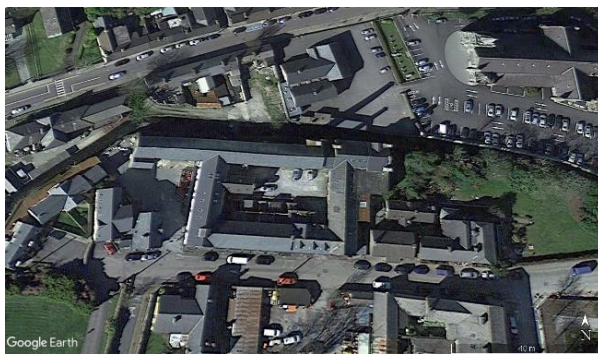
Plate 4.25. Aerial view of Deasy's Brewery in Clonakilty, county Cork. Source: Google Earth.
