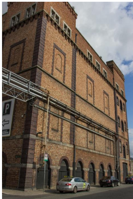
Plate 0.8. Guinness's Robert Street Store, a purpose-built malt store constructed in 1880-4. At the time of its construction it is said to have been both the largest malt store in Europe and also the building with the tallest load-bearing brick walls in the world.
