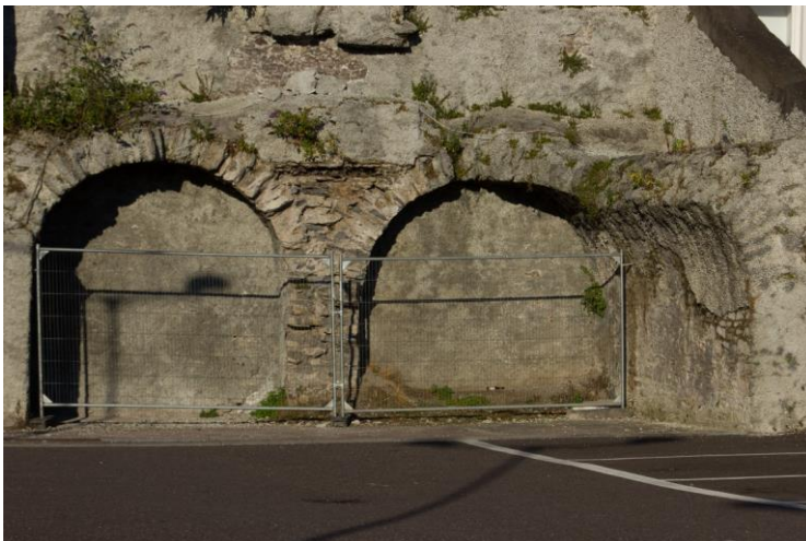
Plate 5.21. Fragmentary remains of former barrel-vaulted spaces, the Southgate Brewery, Cork. These barrel vaults are potentially the remains of early fire-proofed furnaces for brewing coppers.
