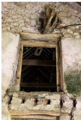
Plate 4.20. Hand-dressed timber sack hoist at the Bantis Brewery, near CloghJordan, county Tipperary.
