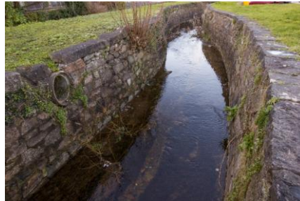
Plate 7.7 Masonry mill race, a canalised tributary of the River Corrib. The Madeira Island Brewery, Galway city.
