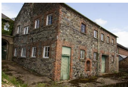
Plate 8.17. Probable stables, the Mill Park Brewery, Enniscorthy, county Wexford.
