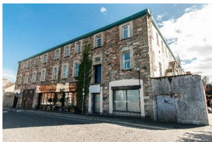
Plate 4.15. Maltings at the Newtownards Brewery, county Down. Note the red-brick scars of the former grain entry point between the two leftmost bays.
