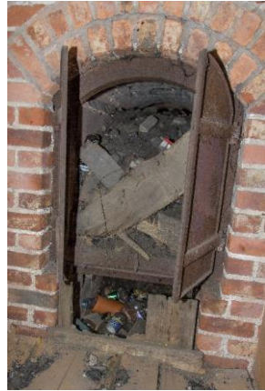
Plate 4.10. Cast-iron malt kiln furnace, the Mill Park Brewery, Enniscorthy.
