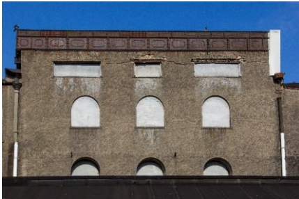
Plate 8.11. Rooftop rivetted cast-iron water tank at Beamish and Crawford, Cork city.
