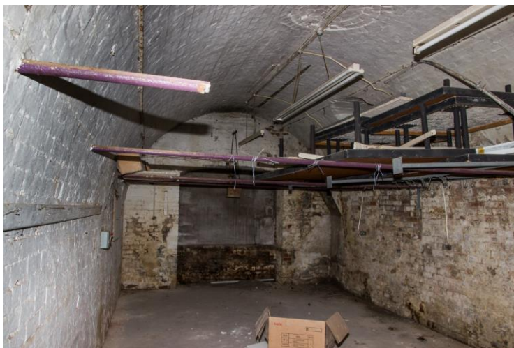
Plate 5.19. Barrel-vaulted furnace arch, the Belfast and Ulster Brewery, Belfast.
