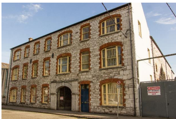
Plate 8.25. The probable brewhouse of Jones and Cowperthwaite's Brewery, Cork city.
