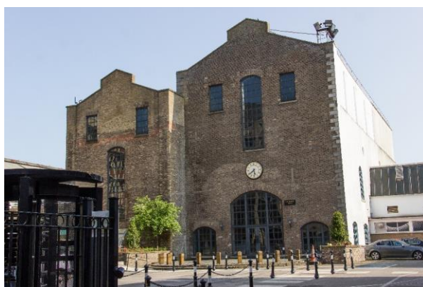
Plate 0.2. Vat houses, dating to the late-18th and early 19th centuries. The sole surviving elements of Guinness's original brewhouse, Brewery No. 1.
