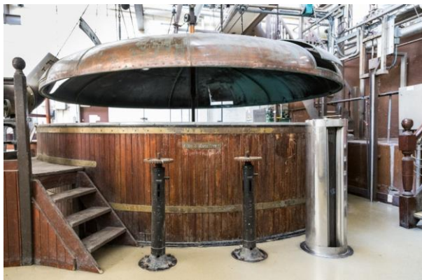
Plate 5.12. Mash tun no. 3, the St. Mary's Brewery, Waterford. The original controls for the Steel's mashing machine can be viewed in the mid-foreground. Their c. 1970 replacements, in aluminium, are located adjacent, to the right.
