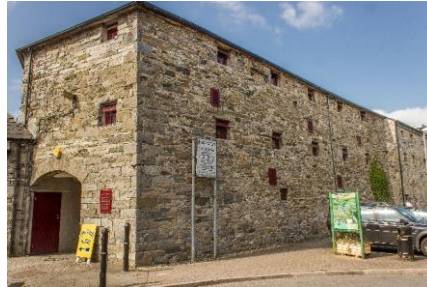
Plate 4.8. Four-storey malting with partially fenestrated ground and first floors, Graham's Brewery, Westport.
