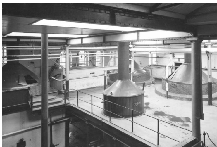
Plate 5.14. Brewing coppers with conical caps at Beamish and Crawford, Cork, in the early 20th century (courtesy Diarmuid Ó Drisceoil).
