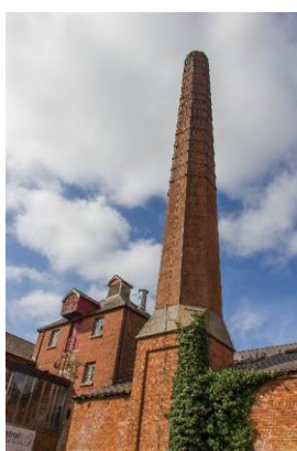
Plate 7.15 Engine house and chimney, dating to the mid-1860s reconstruction. The Cambrickville Brewery, Dundalk, county Louth.
