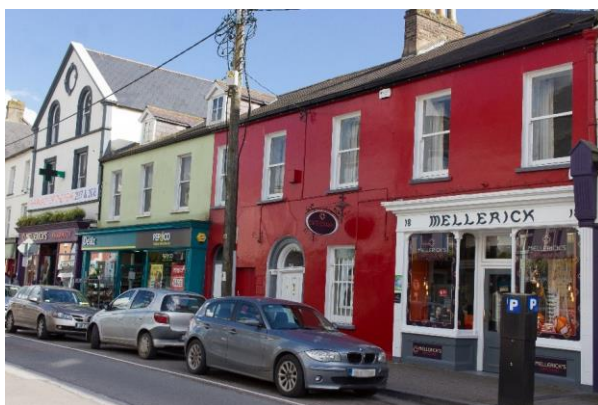
Plate 8.24. The much-altered, two-storey, eight-bay, north range of Walker's Brewery, Fermoy, county Cork.
