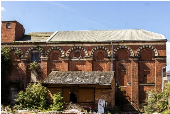
Plate 8.36. Former brewhouse at the Belfast and Ulster Brewery, Belfast. Constructed in 1864-7 in a classical revival style, featuring polychrome brick and sculpted masonry detailing. The mono-pitch building in the mid foreground is a c. 1970s addition.
