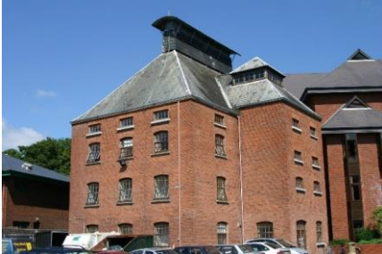
Plate 4.12. Early 20 th century, double-floored malt kiln with ridge ventilator, the Lee Maltings, Cork city. Courtesy C. Rynne.
