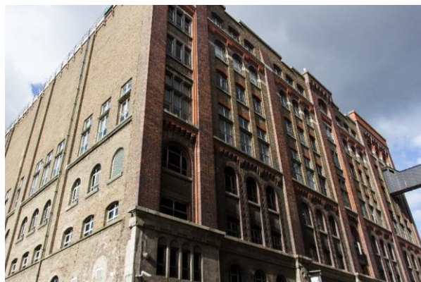
Plate 0.9. Guinness's Market Street Storehouse, viewed from the southwest. The western elevation, on left, is said to be a particularly early examples of a true brick cladding which has been proposed as being the earliest use of such a cladding in Britain or Ireland.
