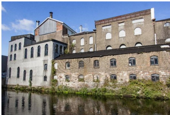
Plate 8.26. The core brewery at Beamish and Crawford, Cork city, viewed from the west. The late-18th and early 19th century brewery buildings comprise the three and four-storey buildings in the background. The 1818 engine house is in the left midground, adjoining it to the right is a two-storey building of unknown purpose, constructed before 1863, while the two-storey mono-pitch buildings in the centre and right midground are cleansing cellars, erected in 1870-1.
