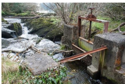
Plate 7.5 Sluice gate at the Dunnamark milling complex, Bantry, county Cork.
