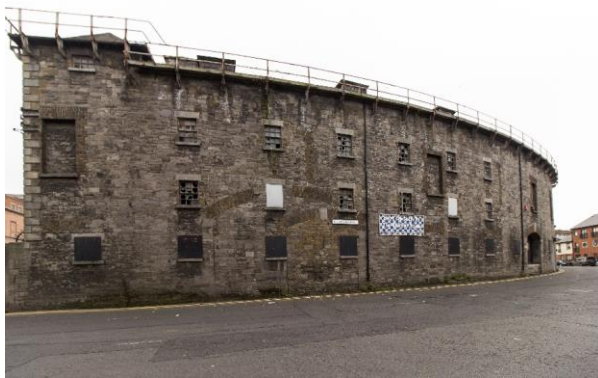
Plate 4.1. Guinness's first purpose-built hop store, constructed on Grand Canal Place in the 1850s or early 1860s.
