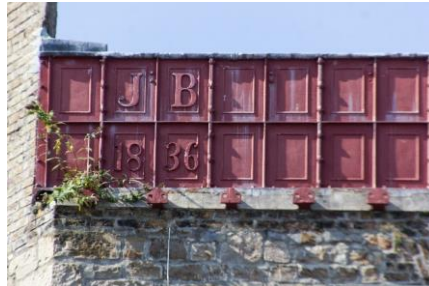
Plate 8.10. Rooftop rivetted cast-iron water tank at the City of Dublin Brewery, originally constructed as a distillery by John Busby in 1836.
