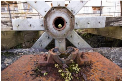
Plate 7.8 Cast-iron bracket for water-wheel axle, the Madeira Island Brewery, Galway city. The water wheel in the background is a recent replica.
