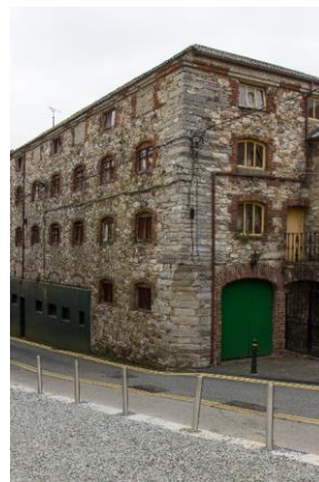
Plate 4.22. Four-storey over semi-basement maltings, Wickham's Gibson's Lane Brewery, Wexford town.
