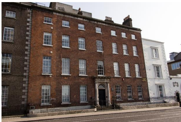
Plate 0.1. The residence of the first Arthur Guinness. Constructed in c. 1770 and overhauled in c. 1870 when it was converted for use as offices.
