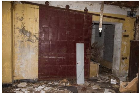
Plate 7.18 Northern set of sliding fire doors in the engine room at the Belfast and Ulster Brewery. They are, potentially, original to the space. The second set was replaced in 1949.
