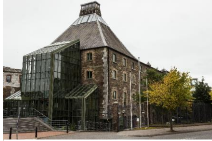
Plate 4.13. Late-1880s century, double-floored malt kiln with ridge ventilator, now glazed. Murphy's Lady's Well Brewery, Cork city.
