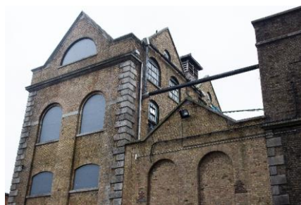
Plate 8.8. The experimental brewery, Guinness, Dublin city. A tower brewery constructed in 1904.
