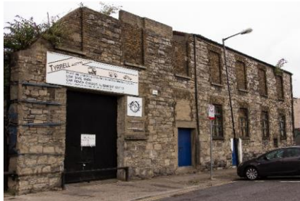
Plate 8.38. Limestone warehouse, Watkins' Brewery, Dublin city.
