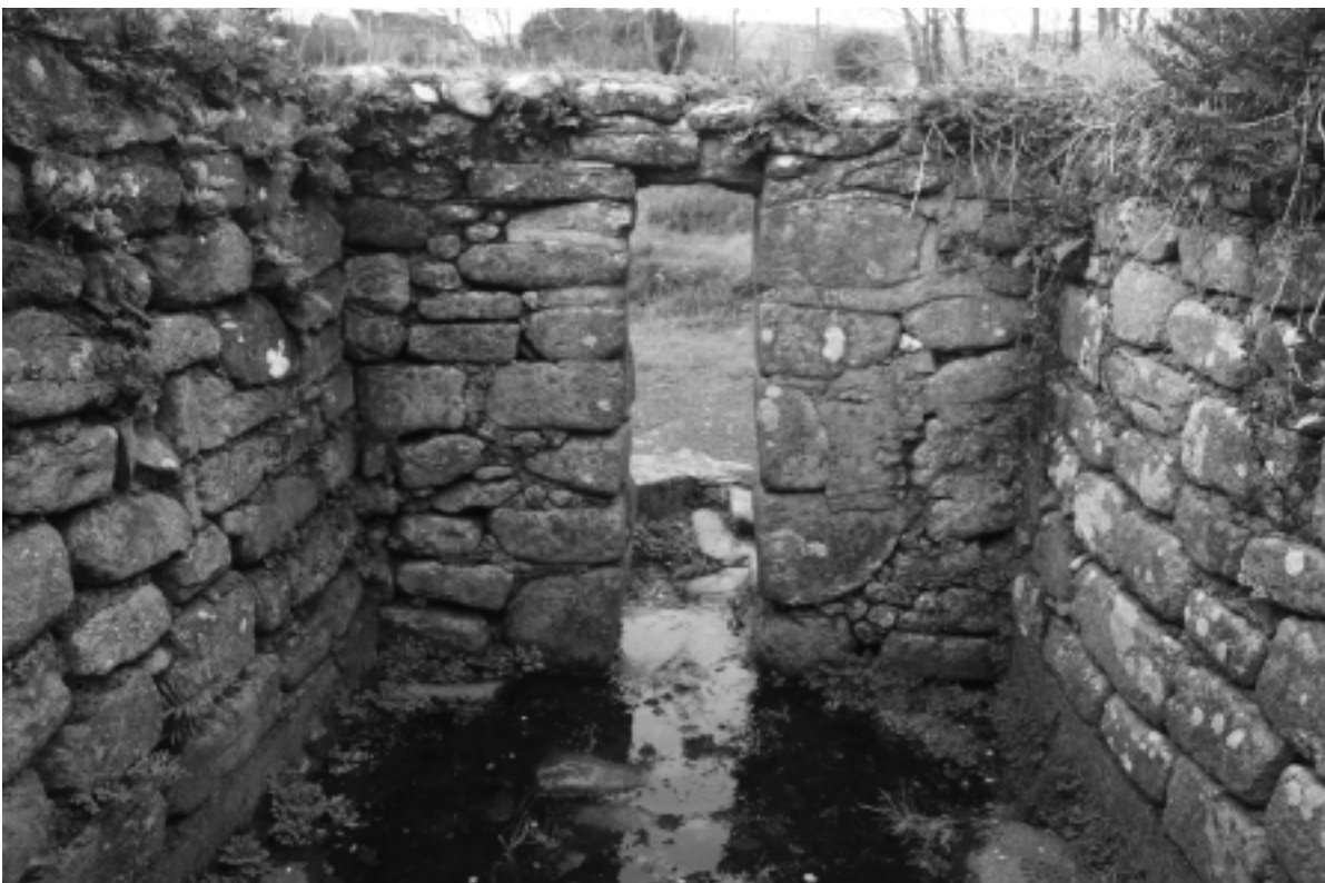
Fig. 10.5 (opposite) St Moling's Well, County Carlow: interior view looking west showing the water flowing through its (rebuilt) flat-headed west door. (© Copyright T. Ó Carragáin)
