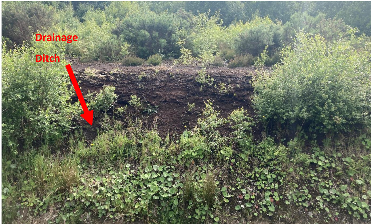
Figure 1.9 Open drainage ditch on a cutaway peatland Lullymore county Kildare Ireland (Photo: author
