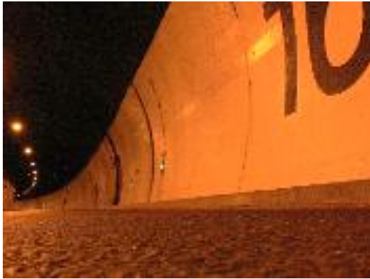
(1) Bored tunnel section
