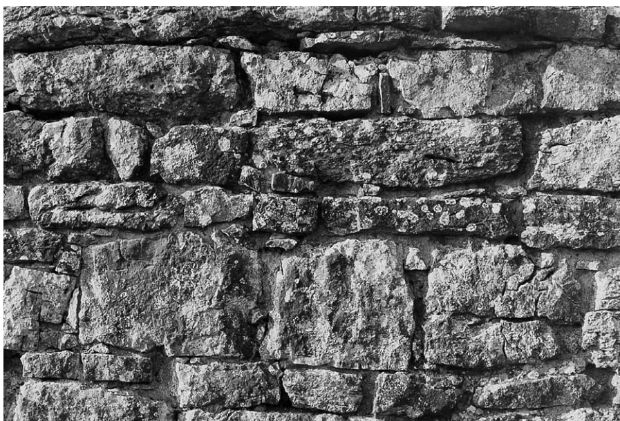
PL. XI—Masonry shot of Killulta, Co. Limerick. Example of the Limerick style.
