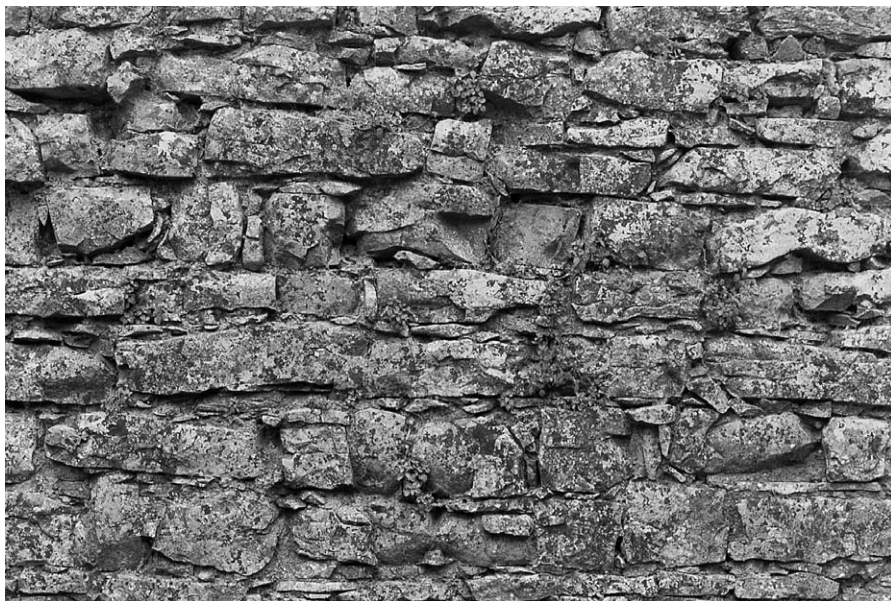
PL. X—Masonry shot of Mungret, Co. Limerick. Example of the Limerick style.
