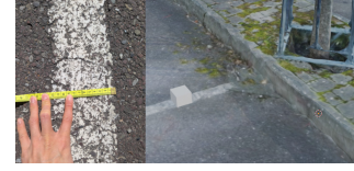
Figure 6. An example of a road marking measurement being used for scale reference.
