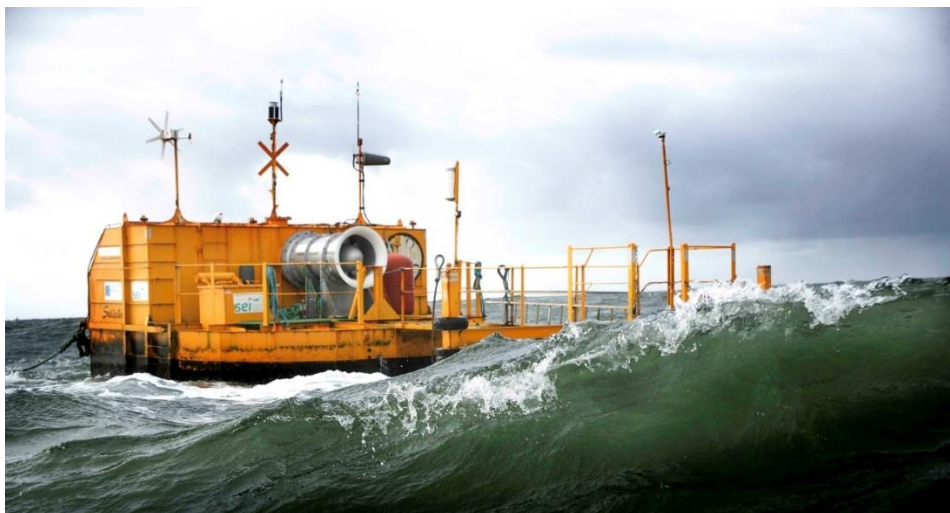
Figure 2.9 The Ocean Energy OE35 Buoy which is an example of a floating oscillating water column (OceanEnergy, 2020).
