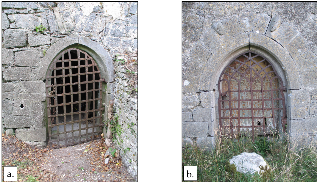
Fig. 2.6 Irish 15 th to 16 th century yetts. a) Clonbrock towerhouse, Co. Galway, b) Donore towerhouse, Co. Westmeath (Both courtesy of Rory Sherlock)
