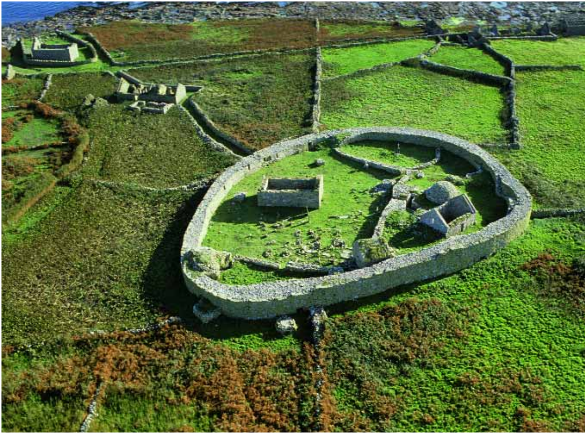
Plate 7 Aerial view of the Cashel (Con Brogan, National Monuments Service)
