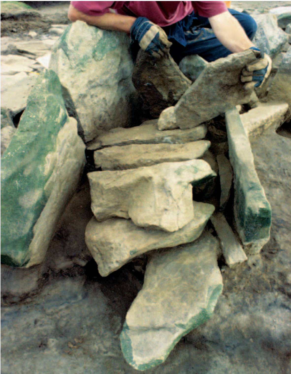
Plate 63 Trahanareear. Details of the wall construction of the cell, with large stones piled flat between outer faces formed by thin edge-set slabs.
