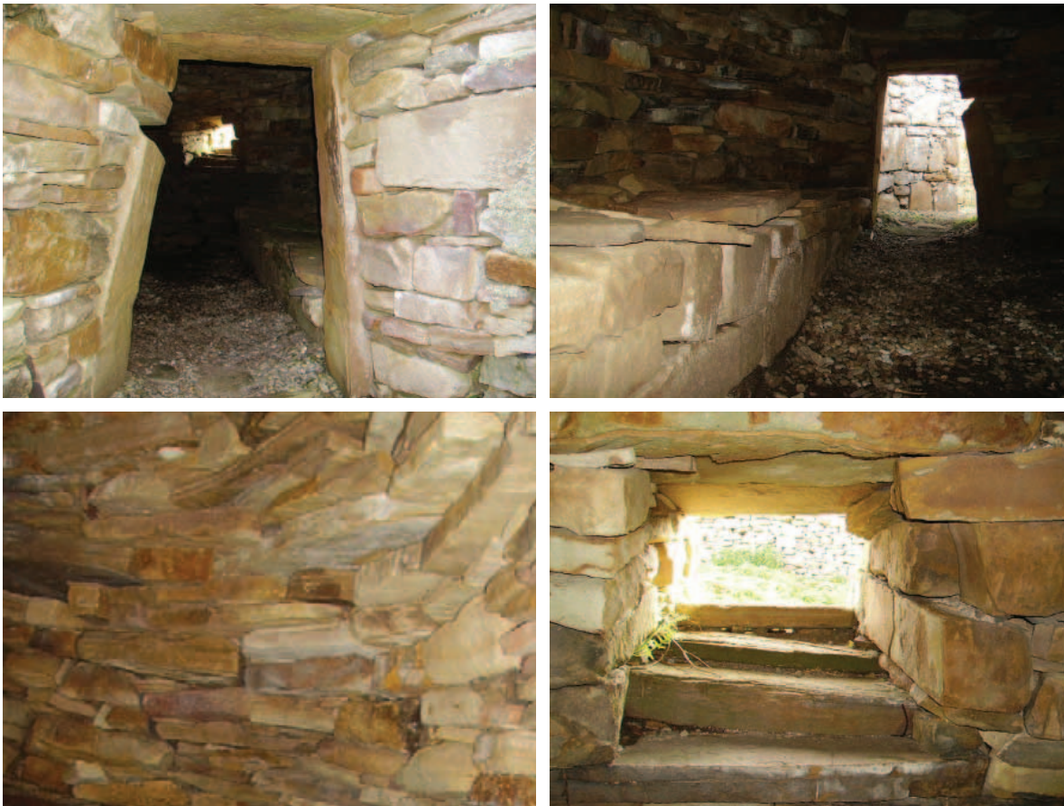
Plate 37 Toorybrenell: details (clockwise from top left) of the doorway, wall bench, window and corbelled roof. The building abuts the corner of the much later Templenatiny and has probably been rebuilt at least once.
