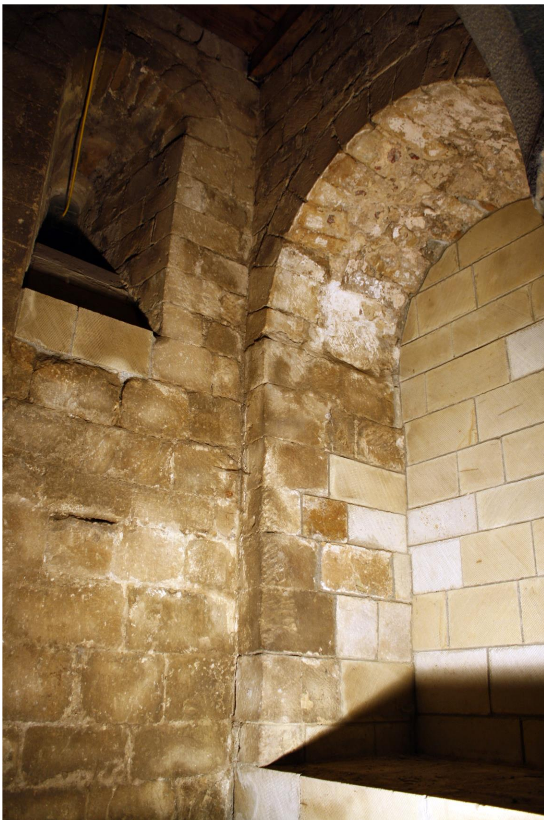
Plate 10 The chamber at the base of the north tower viewed from the doorway at the south showing the now blank niche in the east wall and the window in the north wall (photo: author).
