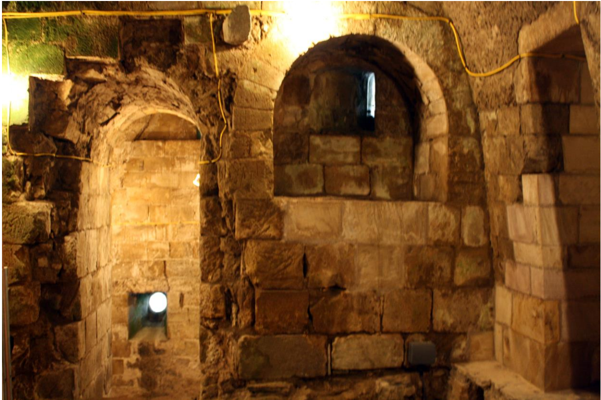
Plate 12 The archway providing access from the upper west chamber to the upper east chamber. The door surround has been removed at some point leaving an irregular aperture on the west side. To the right (south) is one of the pair of niches that flank this archway (photo: author).
