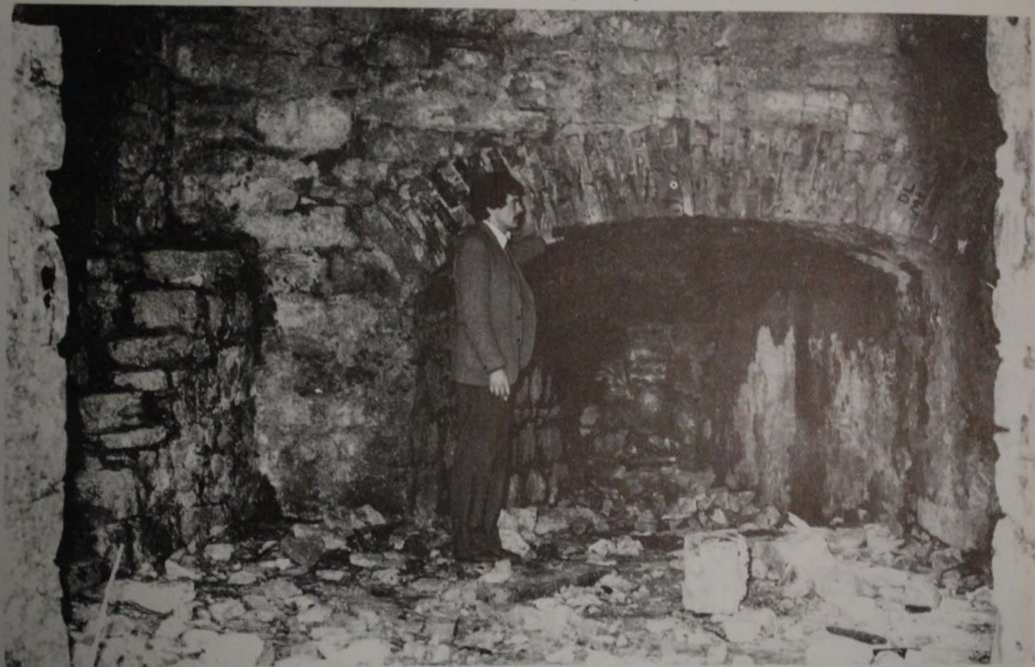
No. 9 Limekiln interior showing steps, ash-pit and arch.
