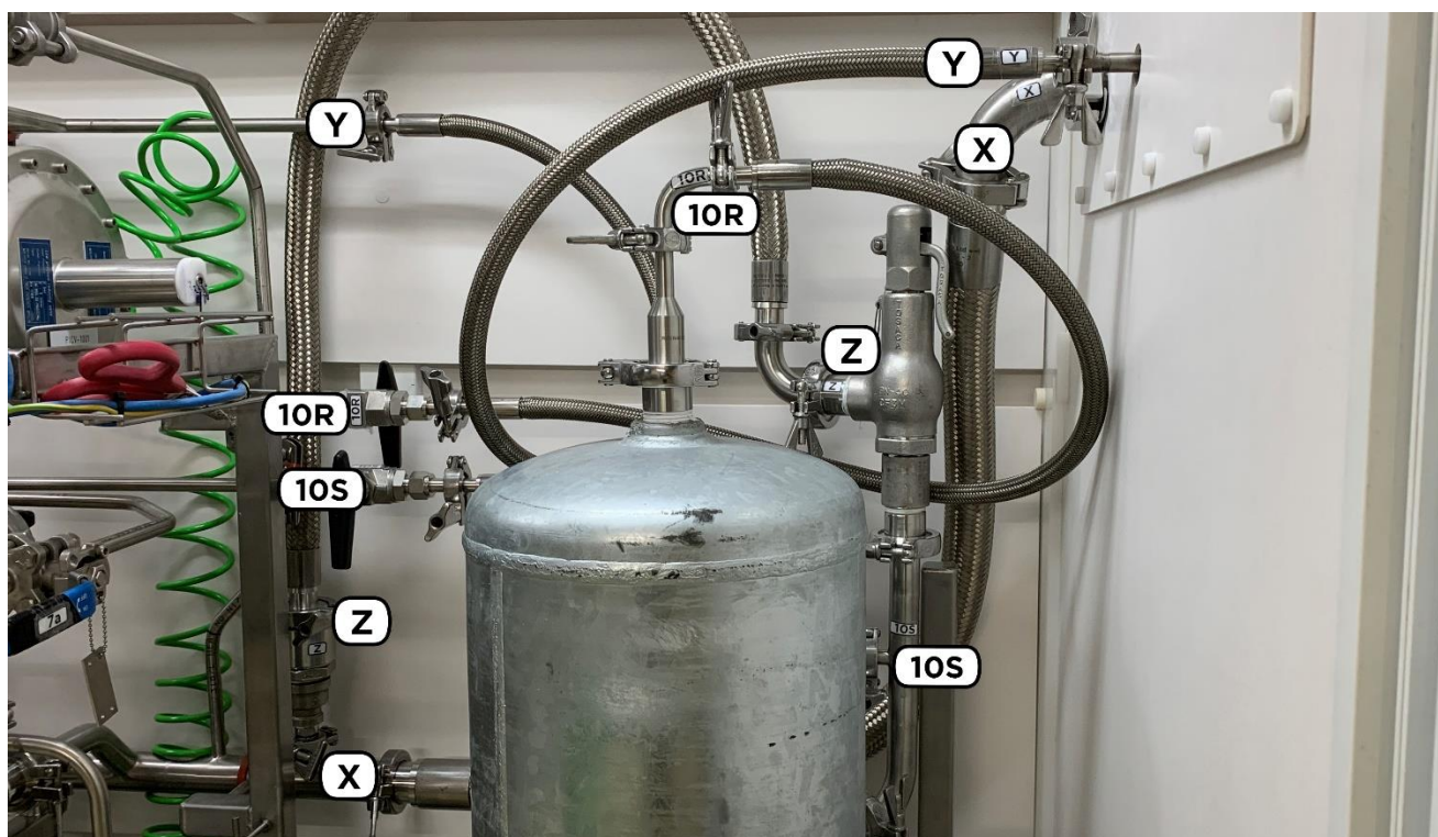
Figure 5: Location of Connection Z and valves/connections 10S and 10R.
