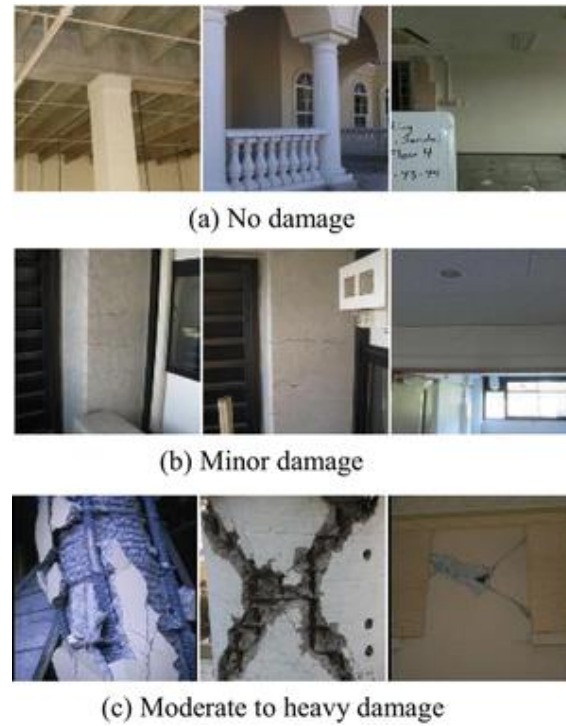
Figure 31-Sample images used in damage level evaluation. (Gao, 2018)
