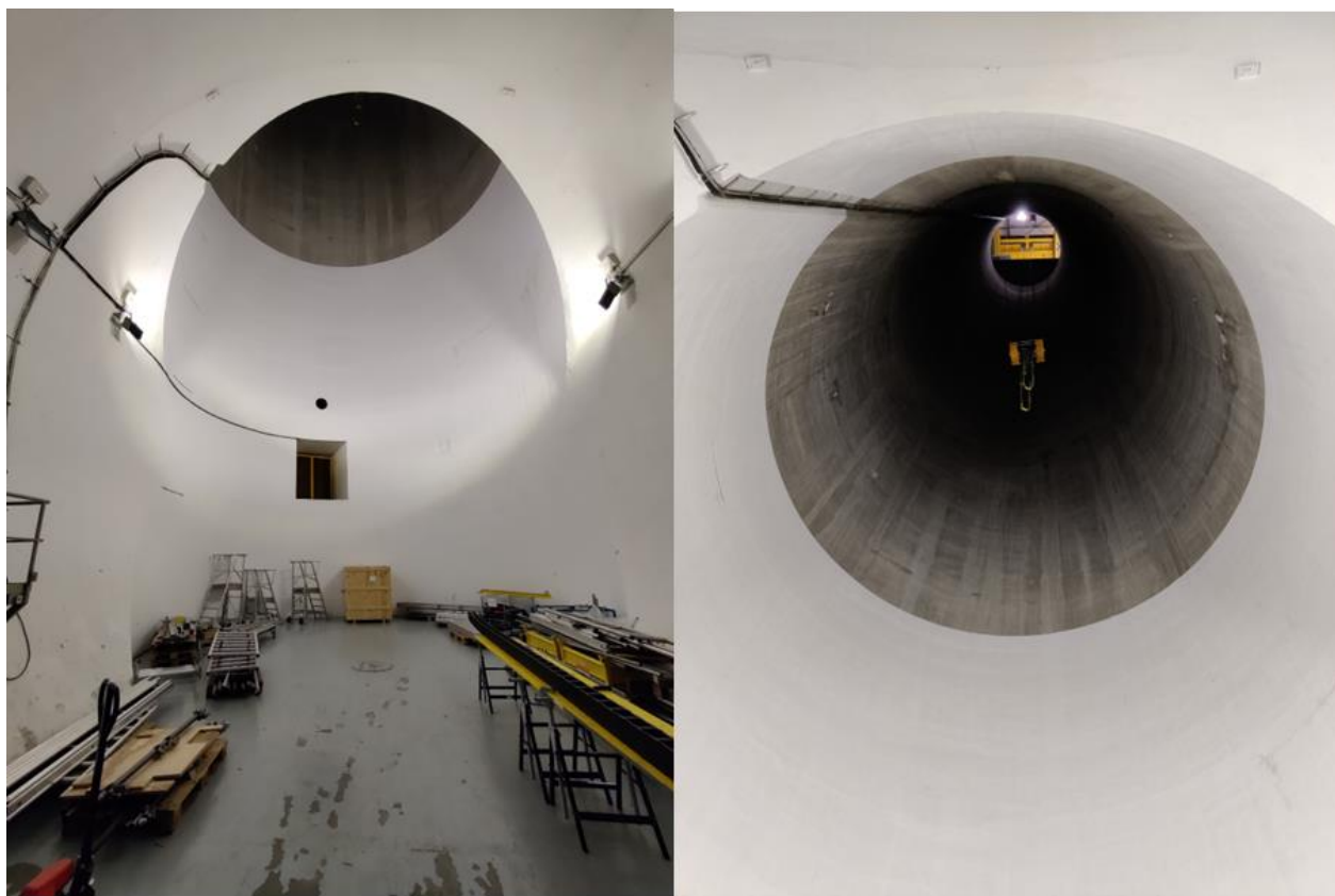
Figure 47 - Images of the Shaft at Point 8 (Images Captured By Author)
