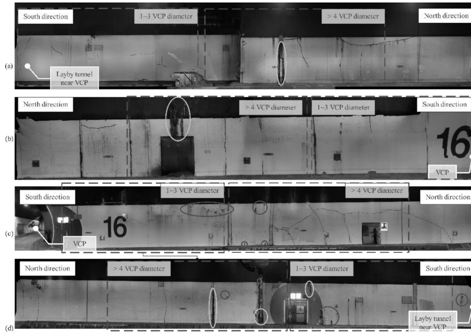
d) Surface Defects Detection
