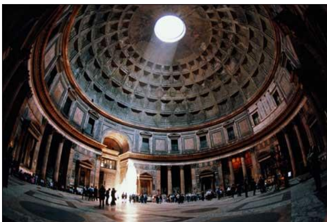
Fig. 2.1 The Pantheon (126 AD): the world's largest unreinforced concrete dome
