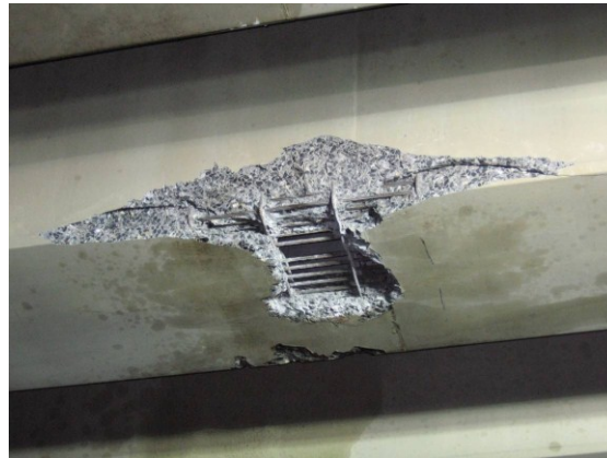
Figure 2 – Photograph of Impact Damage
