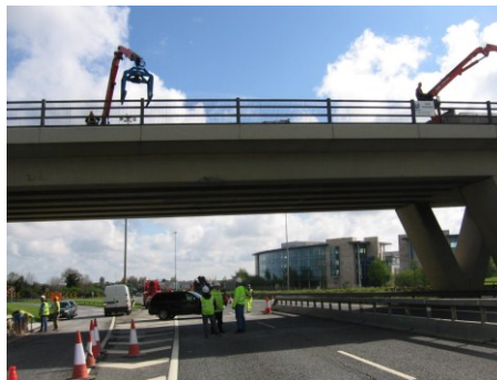
Figure 7 – Removal of Preload
