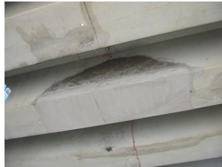
Figure 6 – Repaired Section of Damaged Beam
