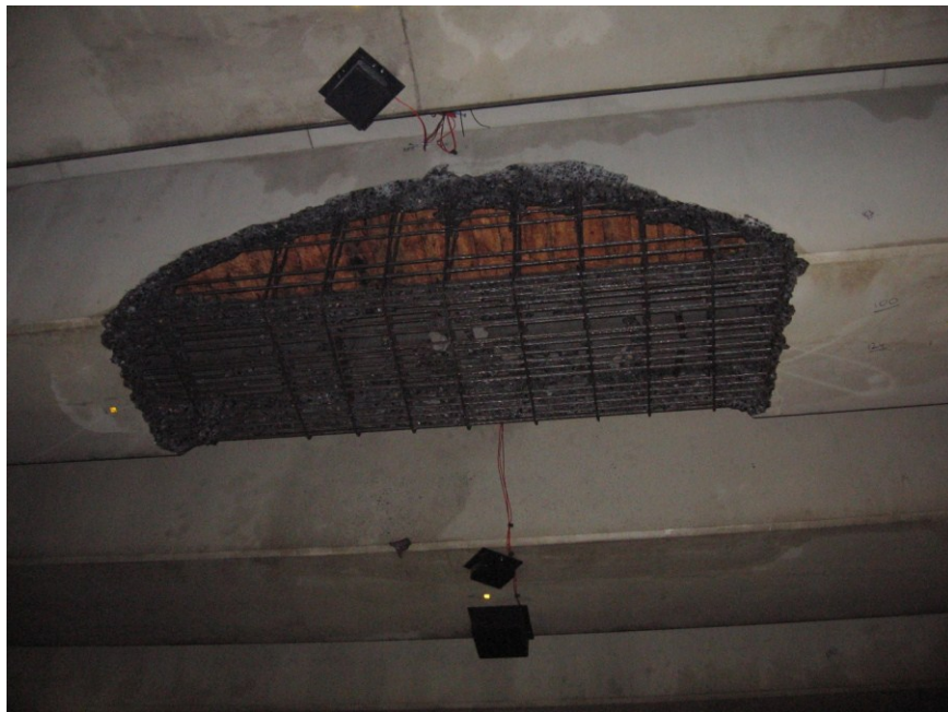
Figure 5 – Removal of Concrete through Hydrodemolition
