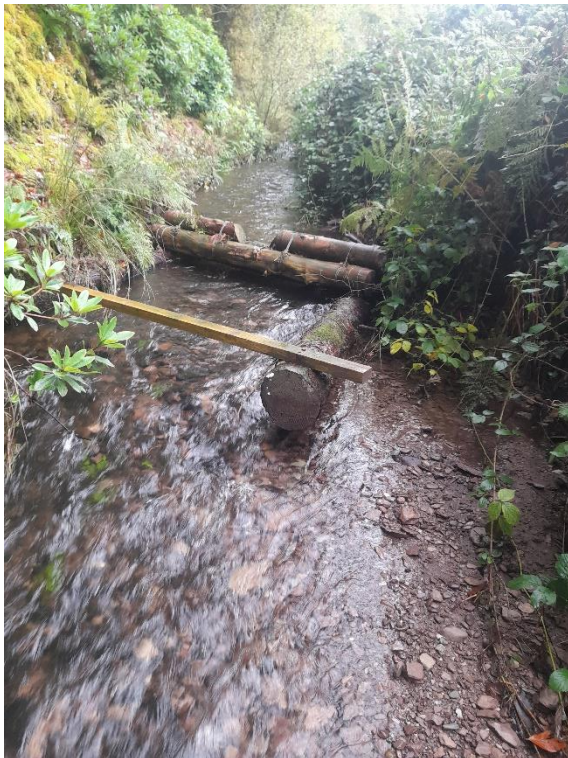
Figure 8 View from downstream of leaky dam displaced approx. 2m downstream during storm event in October 2023
