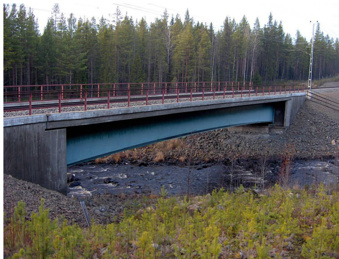
Figure 6.20 Photograph of Skidträsk Bridge [189].
