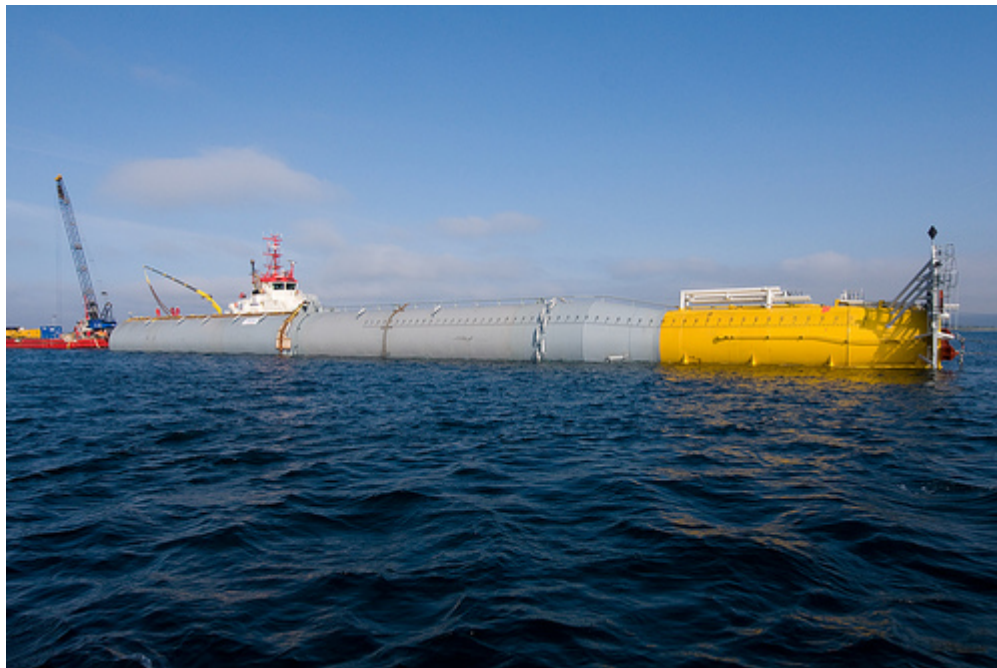
Figure 2-54: Hywind foundation during tow-out
