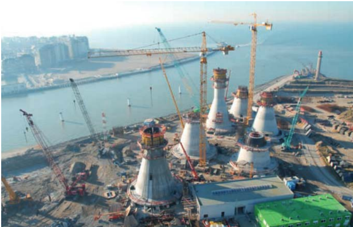
Figure 3-21: Thornton Bank GBS Foundation Port-side construction site
