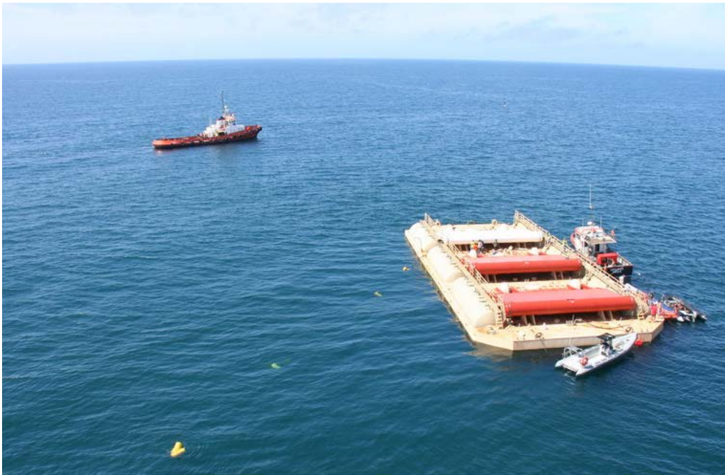
Figure 2-37: Deployment of the 300kW WaveRoller Unit
