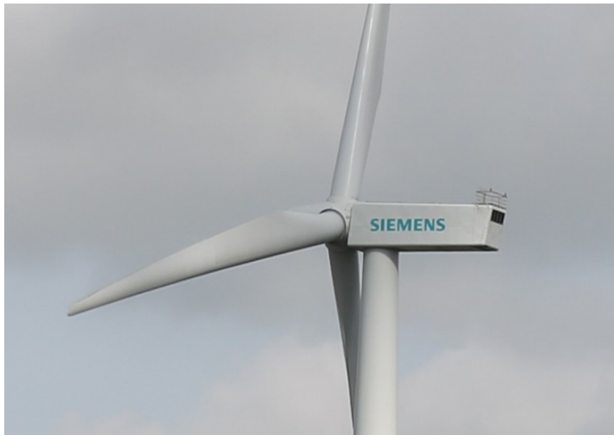
Figure 2-44: The Siemens SWT-3.6-120 3.6MW Turbine
