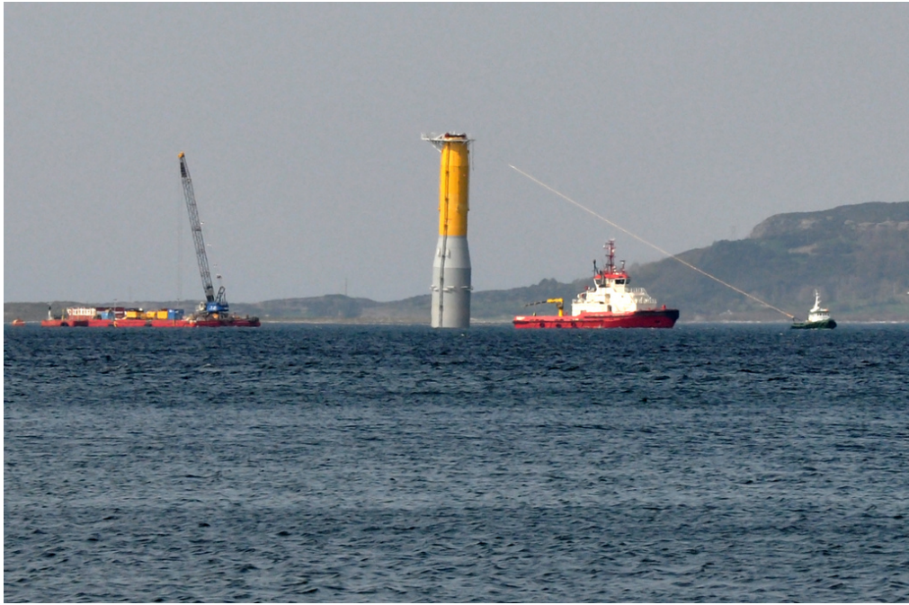
Figure 2-55: Hywind foundation during “upending” procedure
