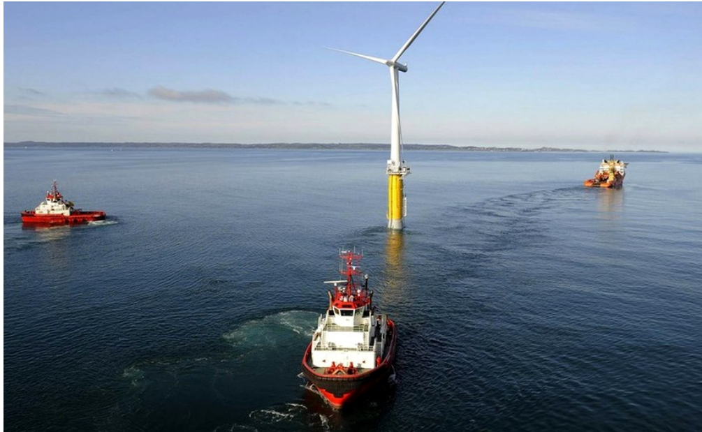
Figure 2-57: Hywind foundation following final installation at Karmoy
