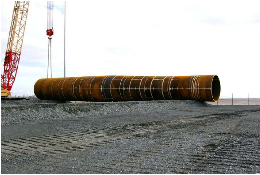
Figure 3-14: Completed Monopile
