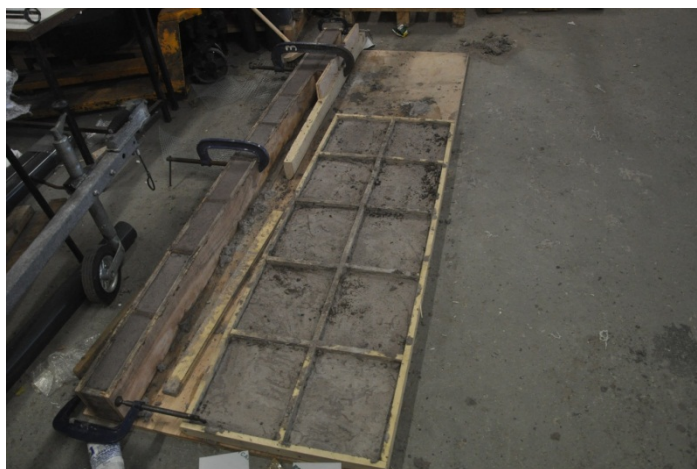
Figure D.3: Casting of concrete ballast blocks
