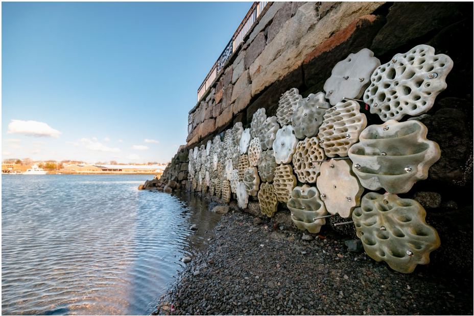
Fig. 5 Living Seawalls panels installed on existing seawalls in East Boston at Condor Street Urban Wild. These modular panels mimic the complexity of natural intertidal habitats, providing refuge for marine organisms
