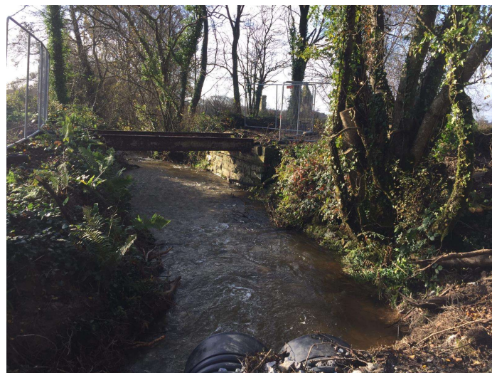
Figure 3. Existing structure on greenway route at Roxborough, showing steel girders and masonry abutments
