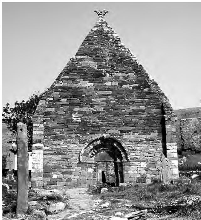
5 Kilmalkedar, Co. Kerry. Note the Romanesque doorway, the otherwise plain façade and the skeuomorphic antae, bargeboards and finial (photo: author).
