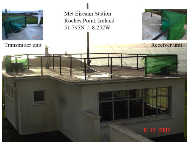
Fig. 7. (Color online) Photograph of the open-path IBBCEA setup on the roof of the Met Éireann weather station at Roches Point (Ireland). The transmitter and receiver units are also shown as insets. The effective cavity length was 6.7 m. The instrument was in this field trial between 29 November and 11 December 2007.
