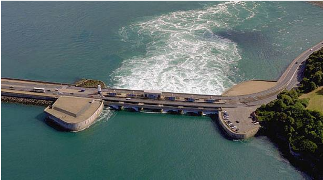
Figure 2.7. La Rance tidal power facility
