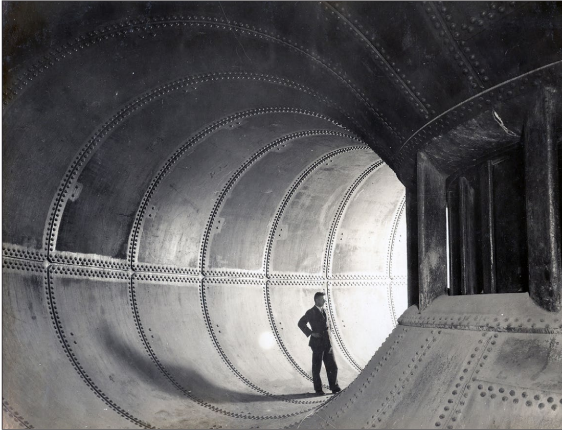
Figure 10: German technician in the turbine at the Ardnacrusha hydro-electric power station (photograph courtesy of ESB Archives).
